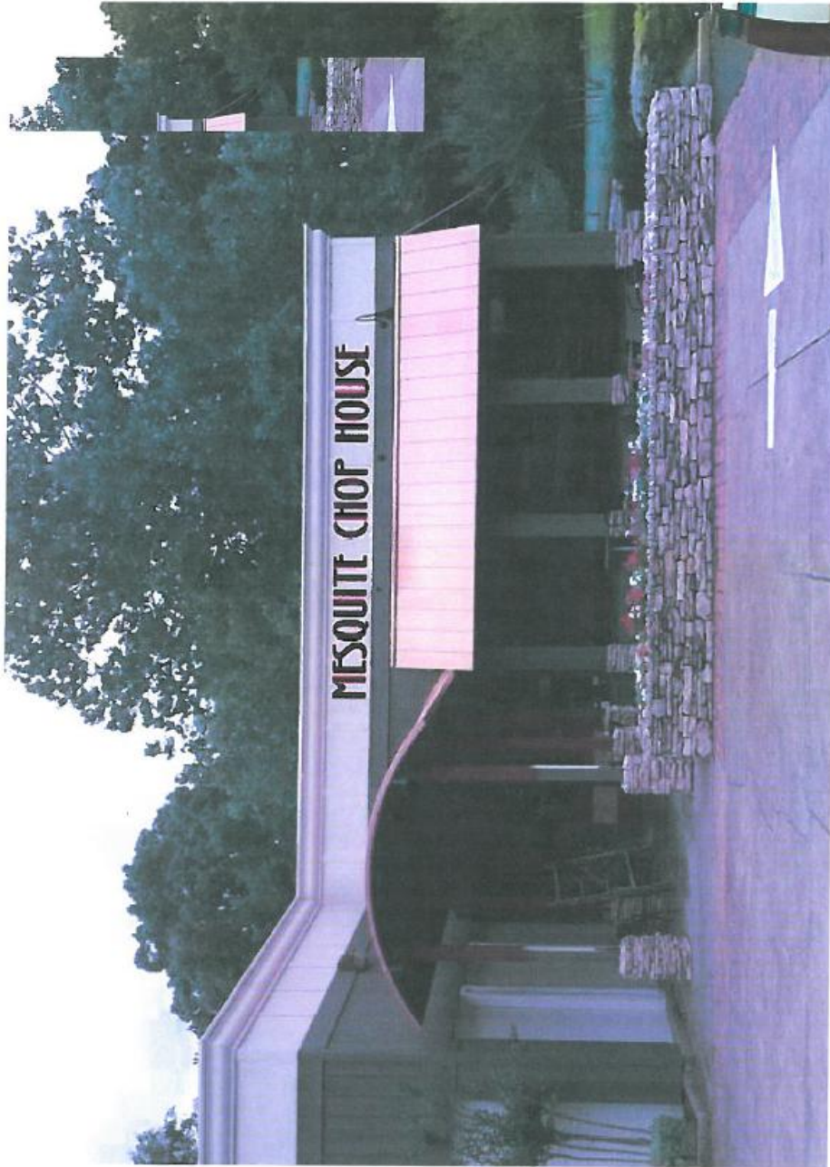
22" reverse channel letters painted black with red border. Letters illuminated by 3 gooseneck lights.
