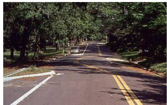
A chicane creates a horizontal deflection in the roadway.
