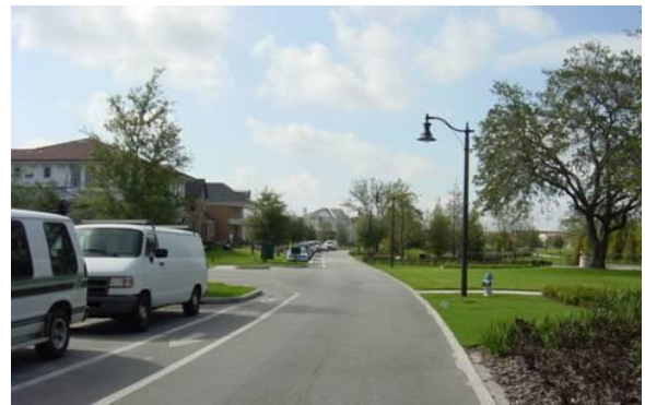
The addition of a bike lane and a parking lane on this street helps to create a narrow travel lane for motorists.
