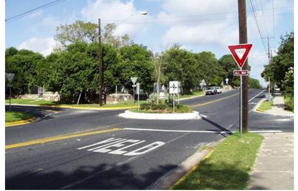
A traffic circle creates a horizontal deflection in the roadway, which causes motorists to slow down as they travel through the intersection.
