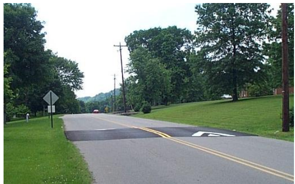
The speed table that may be used in the City of Germantown is 22 feet long and three inches high.
