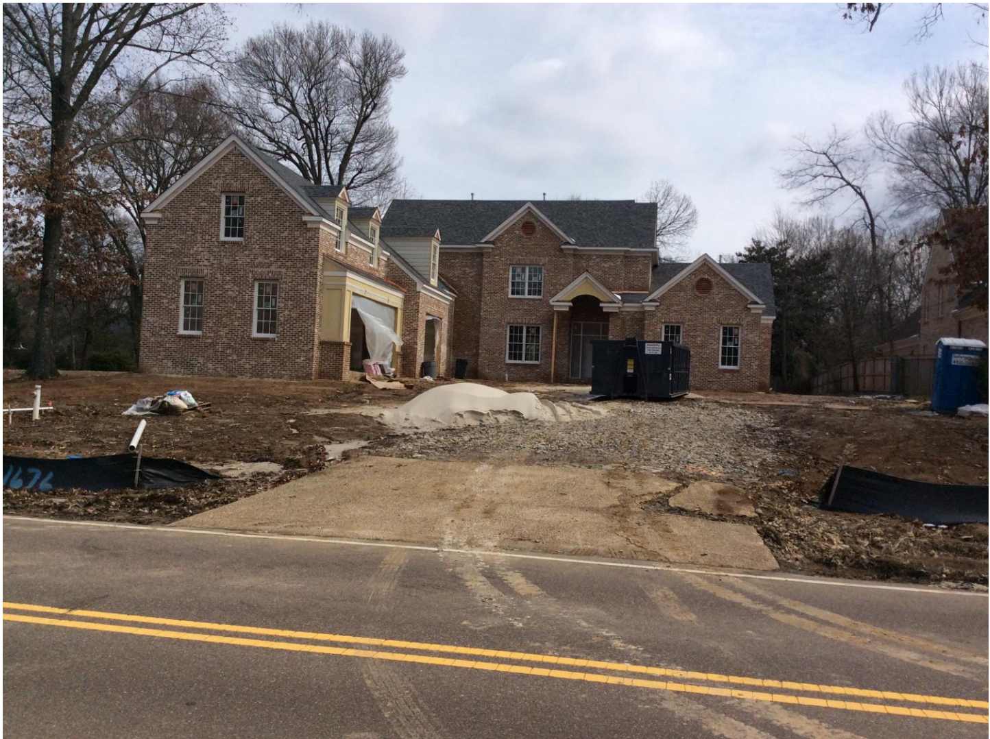
NEW HOUSE CONSTRUCTED ON LOT 1
