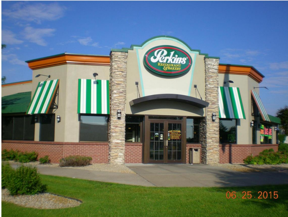
Photo of Another Finished Location with Same features
