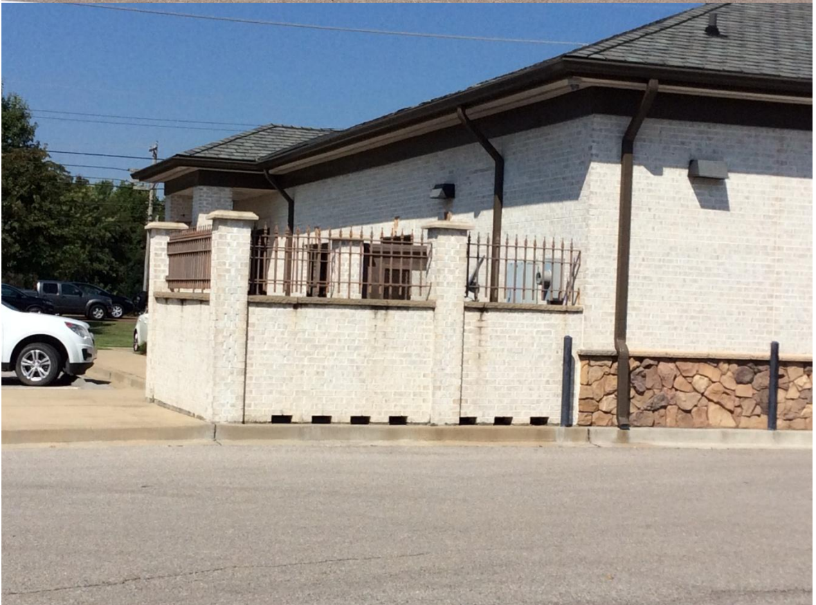
Existing Mechanical Unit Screen Wall
