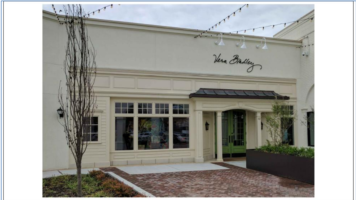
SHOPS AT SADDLE CREEK - GERMANTOWN, TN VERA BRADLEY - EXISTING STOREFRONT ELEVATION SCALE: NONE PROJECT NUMBER: 17158 06/22/17
