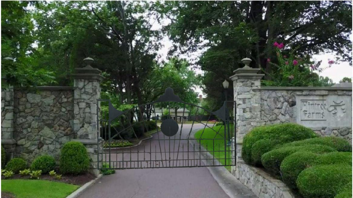
Mock-up Picture of the Aintree entrance with the gate installed
