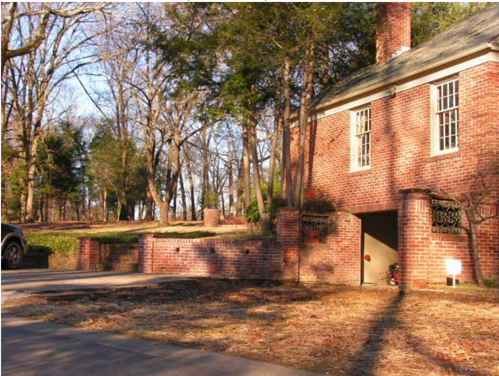
Existing garage and driveway (edge of Radford Ridge Drive along bottom left).
