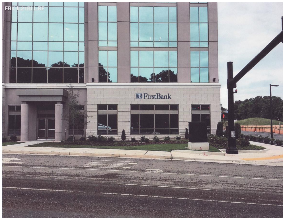
Poplar Avenue Frontage
