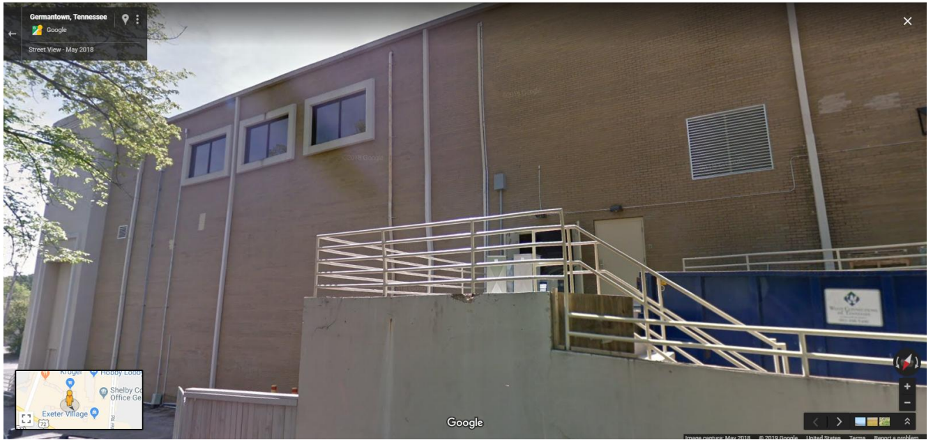
Photos: Existing Rear of Building & Location of Proposed Changes
