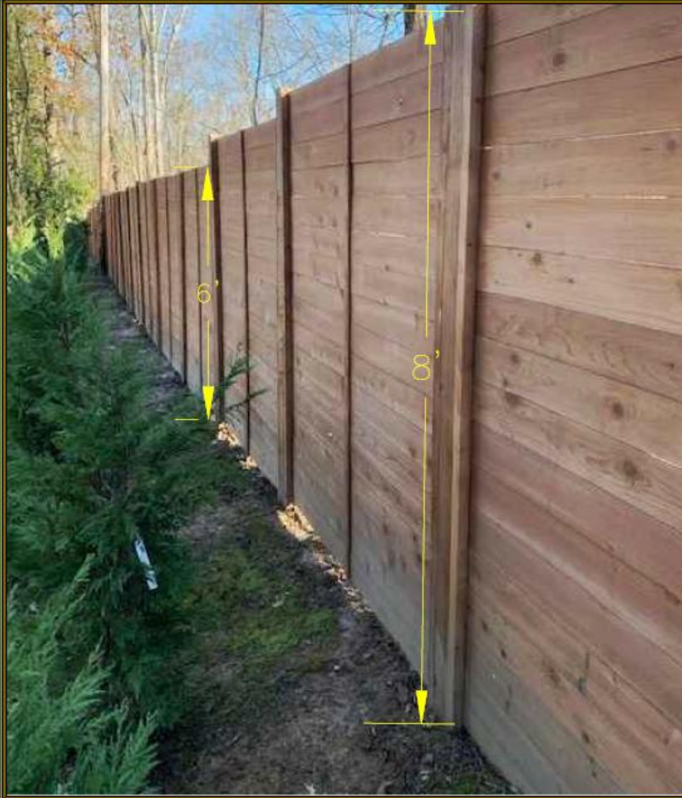
View of fence along east property line
