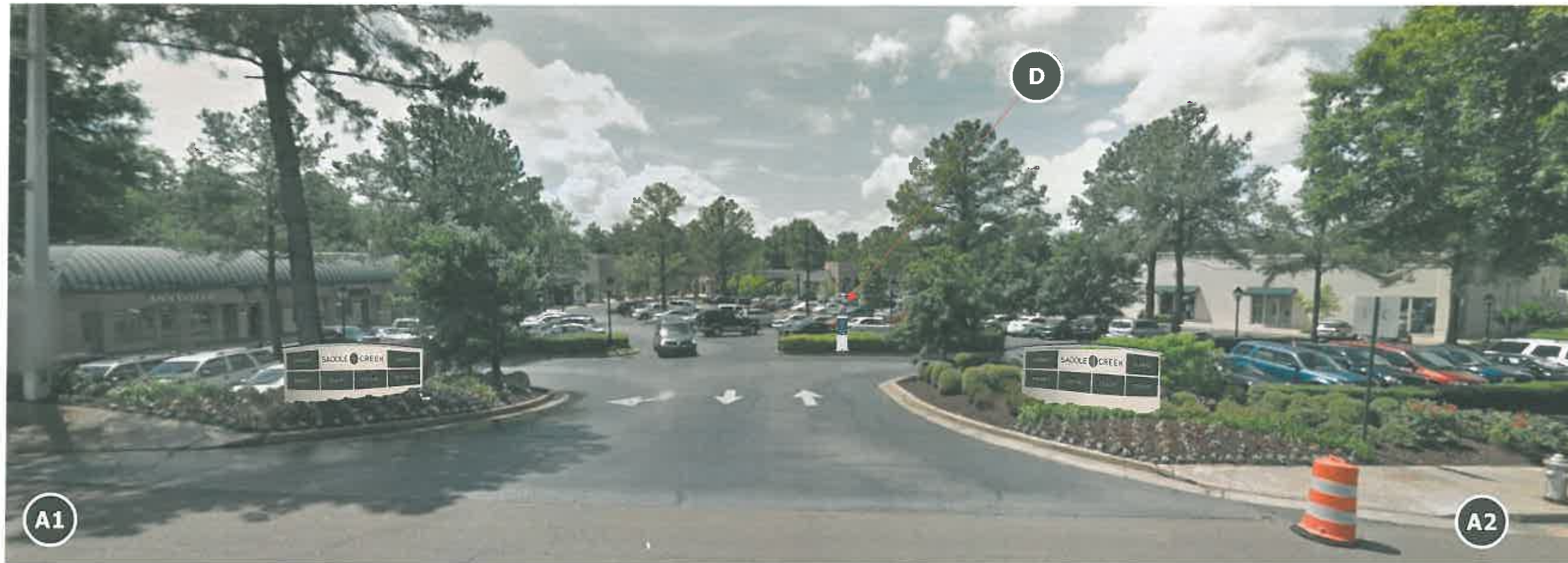
LEFT ENTRANCE TO SHOPPING CENTER
