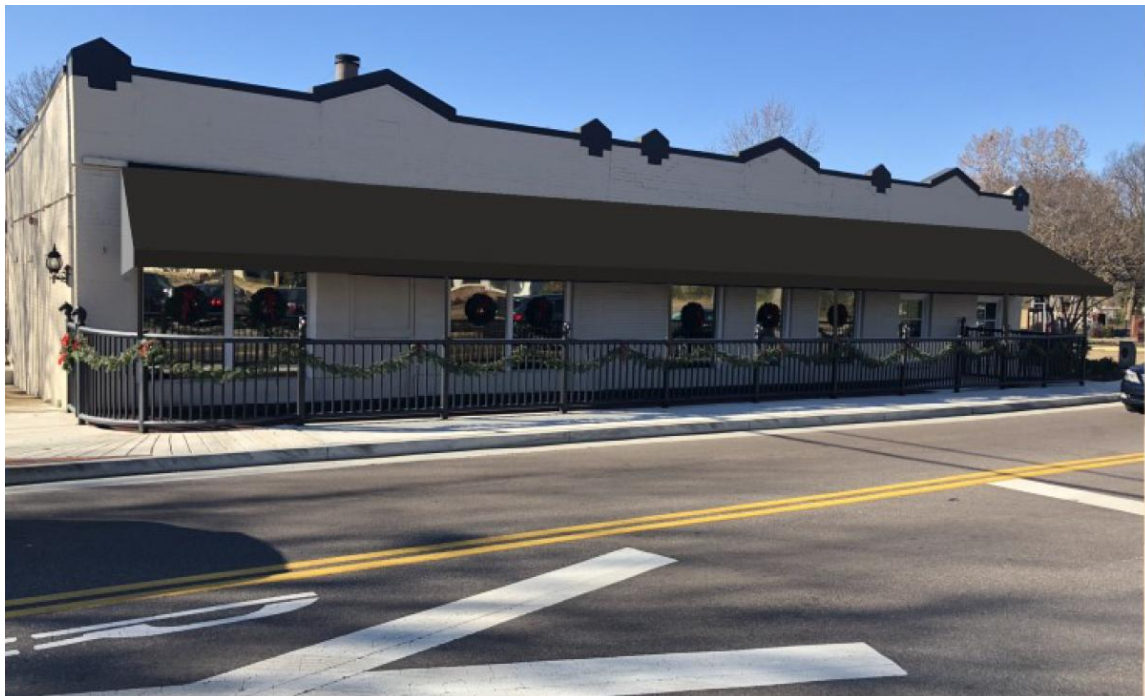
PATIO WITH NEW AWNING THAT COVER ENTIRE AREA
