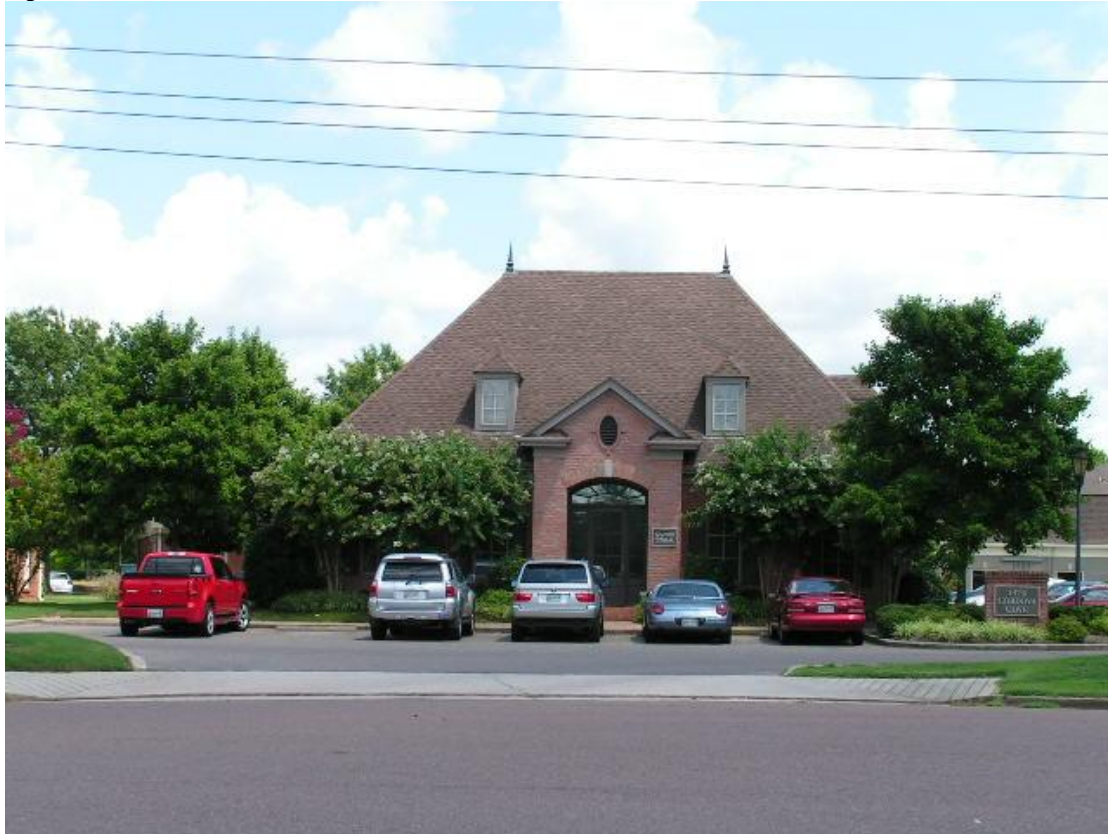
BUILDING TO SOUTH
