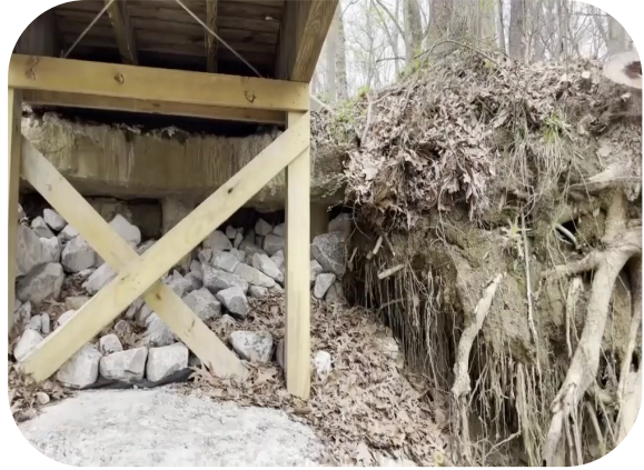
Bob Hailey Access Bridge Replacement
