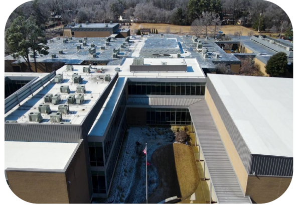
Riverdale Roof Replacement
