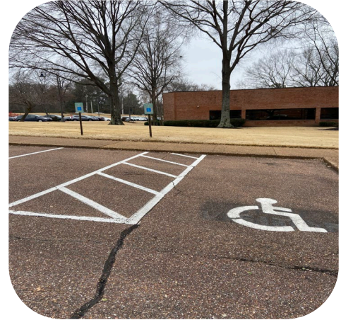
City Hall ADA Parking
