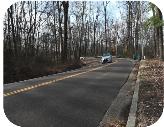
McVay Road Bridge Replacement
