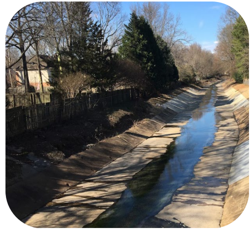
Duntreath Ditch Improvements
