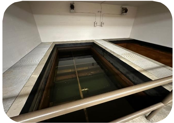
Southern Avenue WTP Filter Bay Refurbishment
