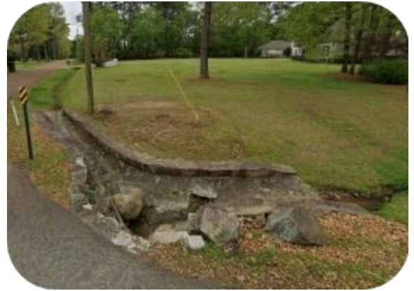
Dogwood Rd & Duntreath Rd Drainage Improvements
