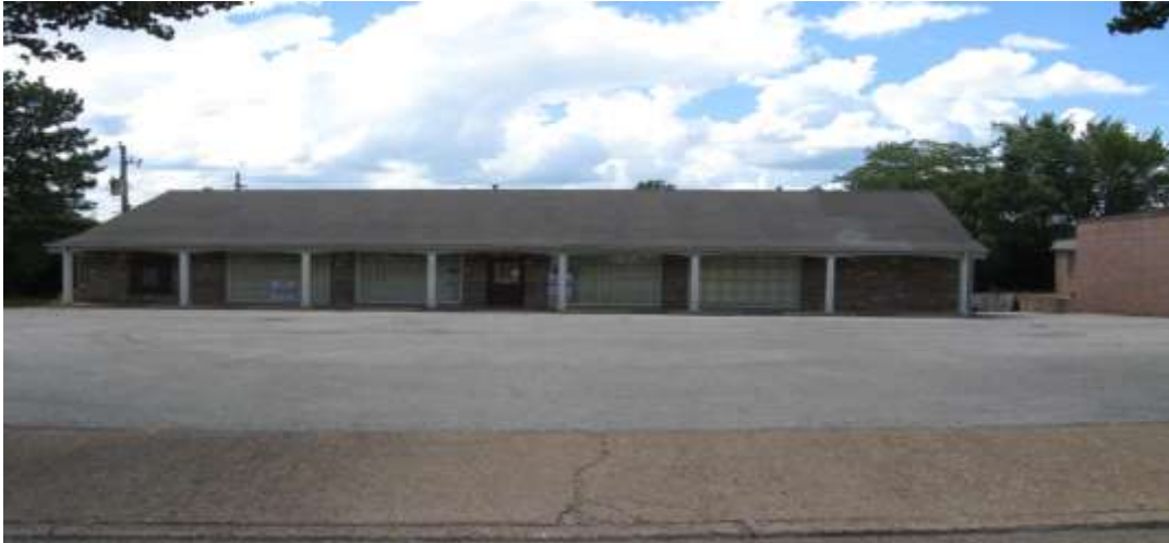
EXISTING BUILDING FAÇADE
