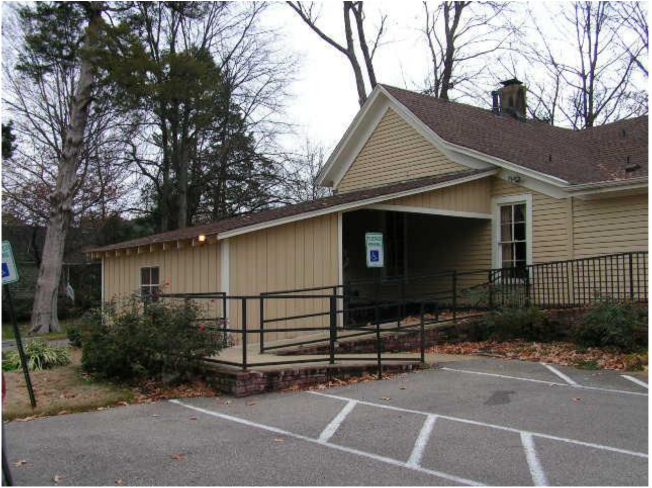
EXISTING CARPORT AND STORAGE BUILDING TO BE DEMOLISHED – view from northwest
