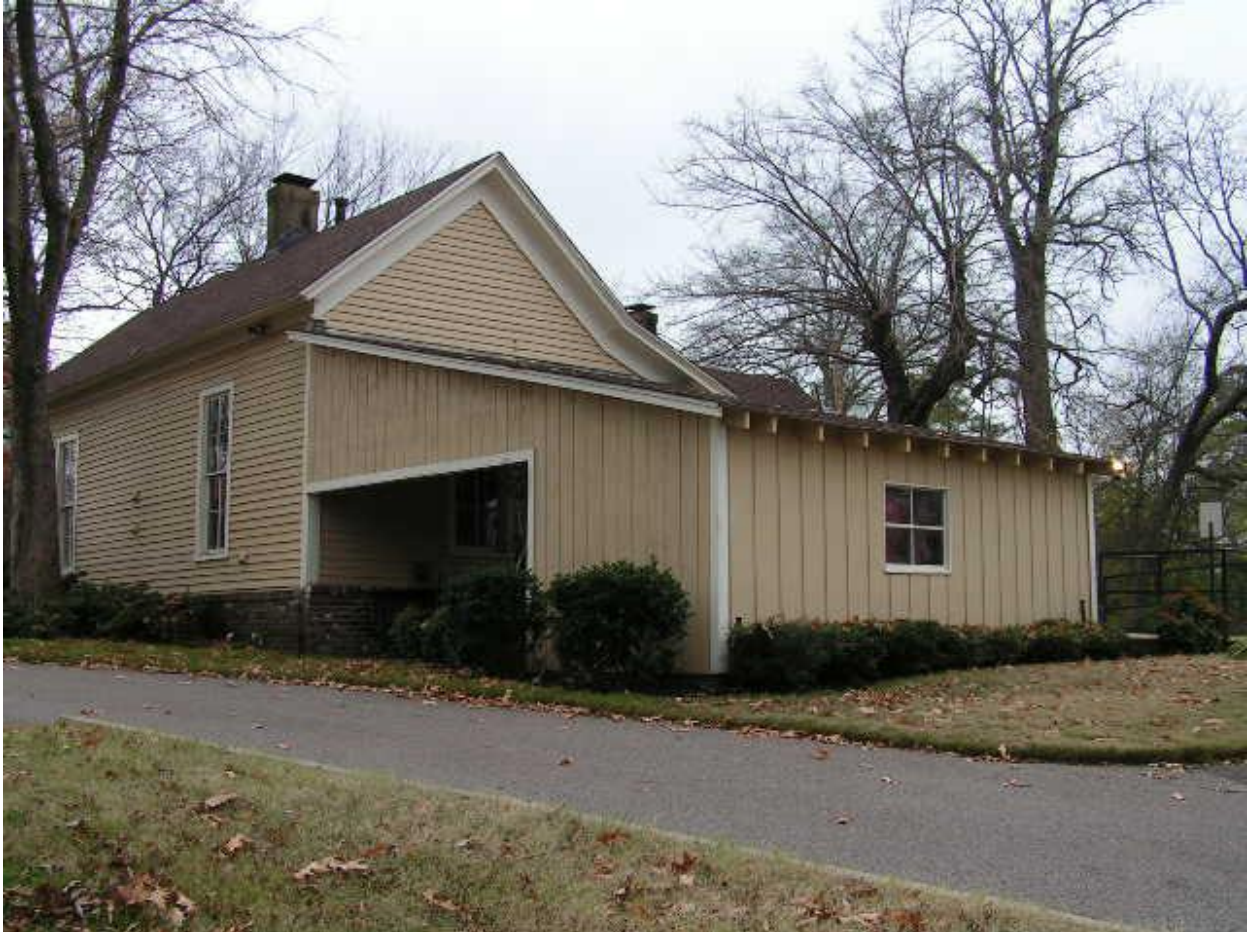
EXISTING CARPORT AND STORAGE BUILDING TO BE DEMOLISHED – view from east
