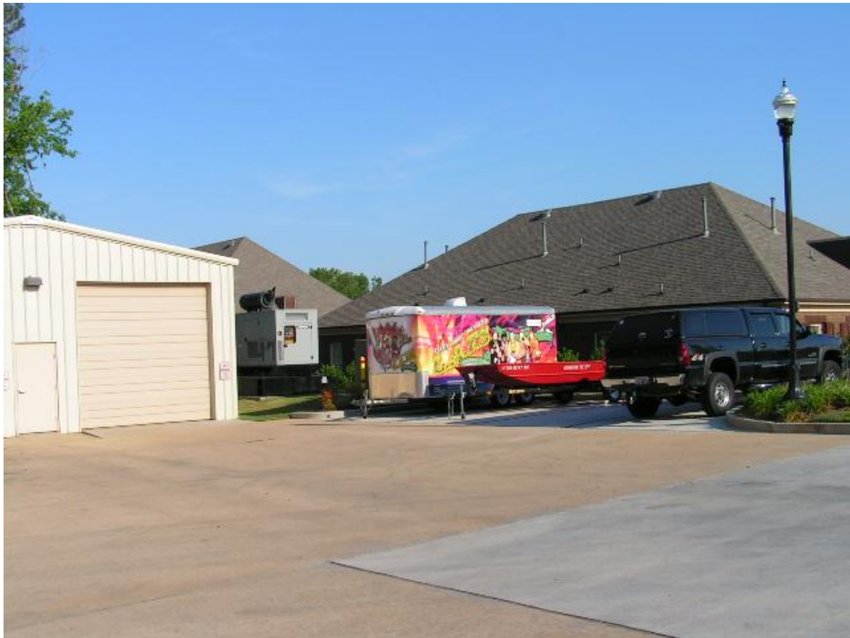
Looking northwest to storage garage, power generator and office buildings along Forest Centre Drive.
